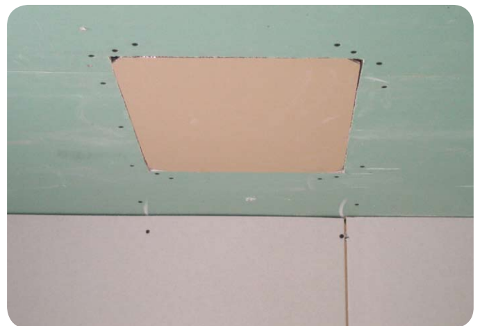
Amina Invisible Loudspeaker installed and ready for plastering.
